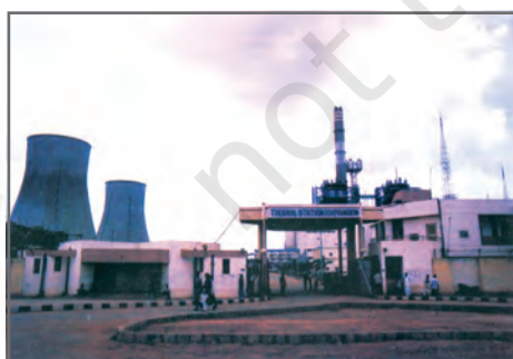
Fig 3.10: A view of a Thermal Power Station
