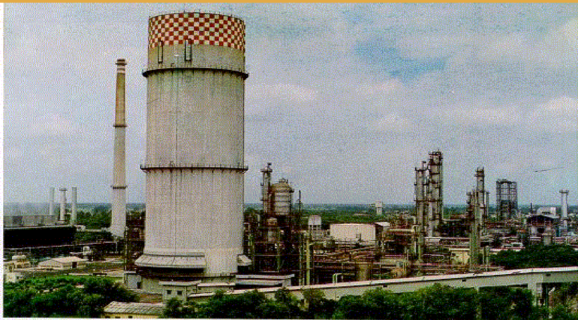
Urea Plant of Indo Gulf at Jagdishpur (Sultanpur, U.P.).
