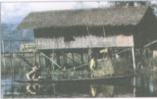
Use of stilts for raised floor above flood level
