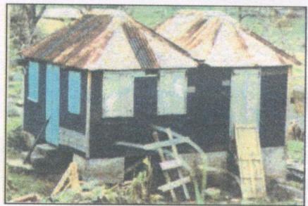
If natural elevational not available construction on stilts or on artificially raised earth mounds
