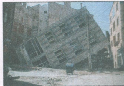
Tilting of building due to liquefaction (Adapazari Turkey 1999)
