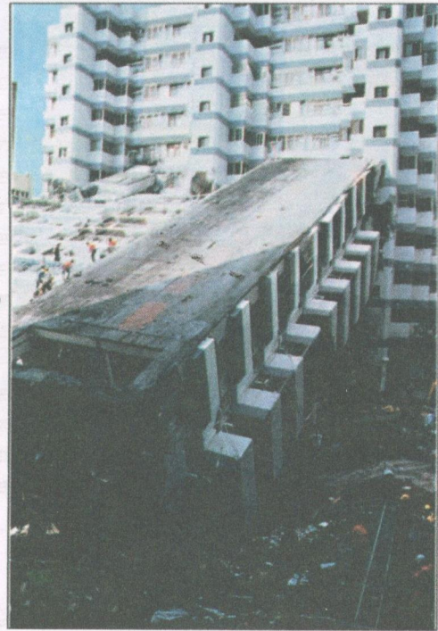
The building has tilted as a result of column failure & as partly damaged the nearby building (Taiwan 1999). (By Bachmann H., Seismic Concep-
