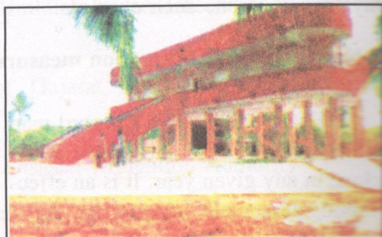
Multi-purpose Cyclone Shelters of suitable designs have been constructed in vulnerable locations of coastal Orissa.
