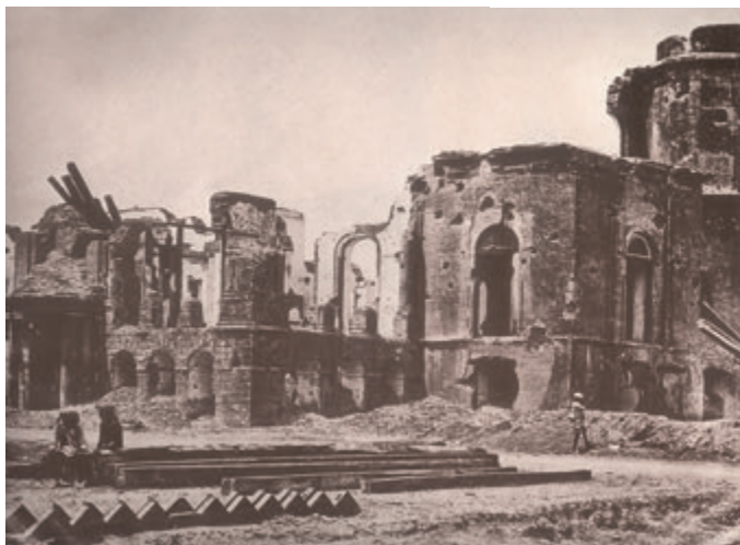
Fig. 17 – Ruins of the Residency in Lucknow
