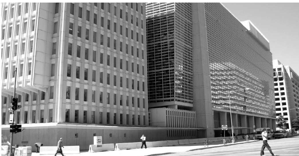
Fig. 4.7 World Bank Headquarters at Washington
