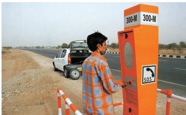
Fig. 7.10 : Emergency call box on NH-8
