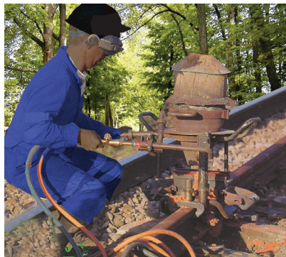
Figure 3.11 Thermit process for joining railway tracks
