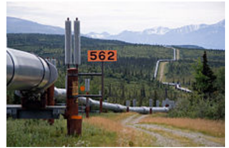
Trans-Alaska Pipeline for crude oil
