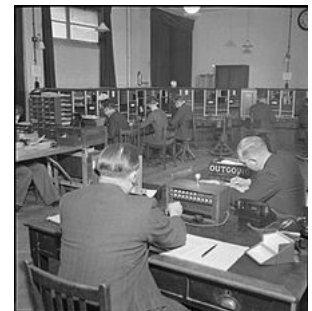
Testing telephone lines in London in 1945.
