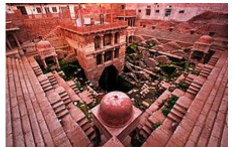
Toor Ji Ki Bawari, stepped well, Jodhpur
