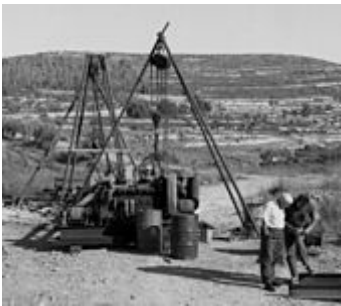
Water well drilling in Ein Hemed, near Jerusalem circa 1964
