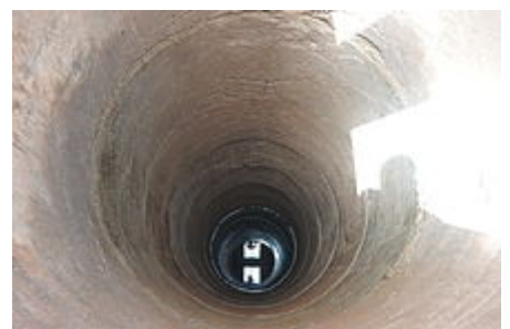
View into a hand-dug well cased with concrete rings; Ouelessebouyou, Mali.
