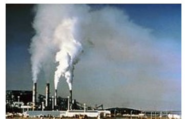
Before flue-gas desulfurization was installed, the air-polluting emissions from this power plant in New Mexico contained excessive amounts of sulfur dioxide
