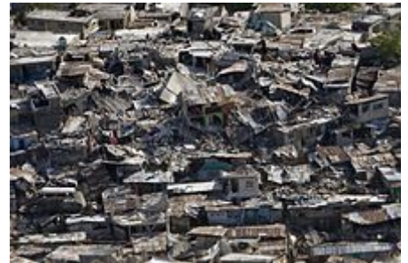
Damaged buildings in Port-au-Prince, Haiti, January 2010.
