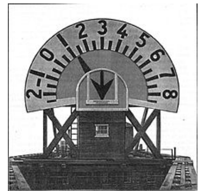
Tidal Indicator, Delaware River, Delaware c. 1897. At the time shown in the figure, the tide is 1\frac{1}{4} feet above mean low water and is still falling, as indicated by pointing of the arrow. Indicator is powered by system of pulleys, cables and a float. (Report Of The Superintendent Of The Coast & Geodetic Survey Showing The Progress Of The Work During The Fiscal Year Ending With June 1897 (p. 483))
