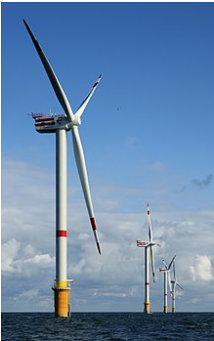
Wind is a natural resource that can be used to generate electricity as with these 5MW wind turbines in Thorntonbank Wind Farm 28 km (17 mi) off the coast of Belgium
