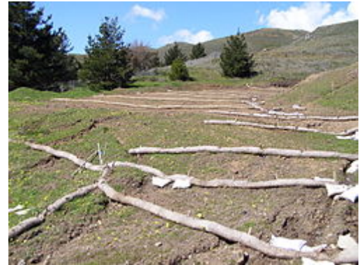
Erosion barriers on disturbed slope, Marin County, California
