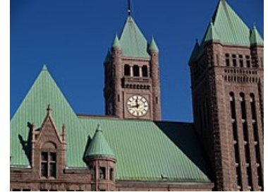
Copper roof on the Minneapolis City Hall, coated with patina
