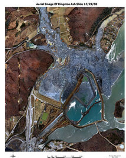
Aerial photograph of the site of the Kingston Fossil Plant coal fly ash slurry spill taken the day after the event
