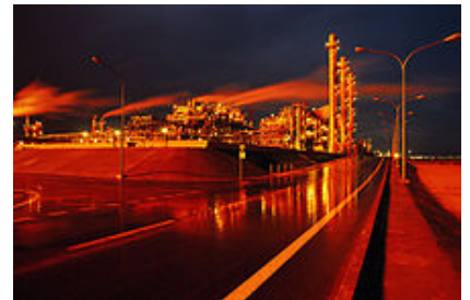
An oil refinery in Mina Al Ahmadi, Kuwait.
