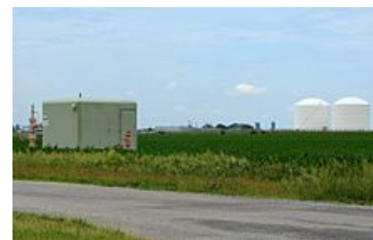
Peoples Gas Manlove Field natural gas storage area in Newcomb Township, Champaign County Illinois. In the foreground (left) is one of the numerous wells for the underground storage area, with an LNG plant, and above ground storage tanks are in the background (right).
