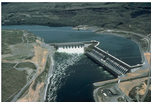
Chief Joseph Dam near Bridgeport, Washington, U.S. , is a major run-of-the-river station without a sizeable reservoir
