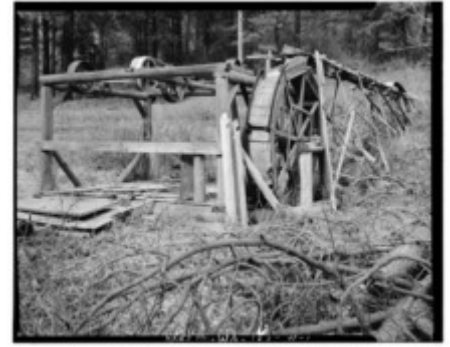
Directly water-powered ore mill, late nineteenth century
