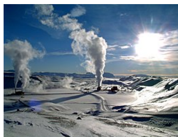
Krafla , a geothermal power station in Iceland
