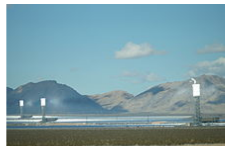
The 377 MW Ivanpah Solar Electric Generating System with all three towers under load, Feb 2014. Taken from I-15.
