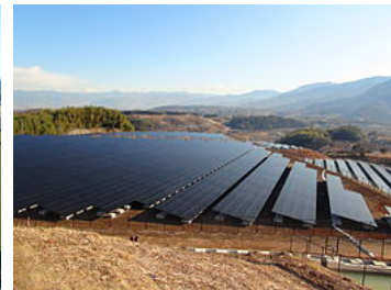
Komekurayama photovoltaic power station in Kofu , Japan
