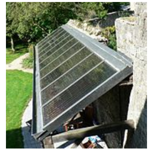
Solar water heaters facing the Sun to maximize gain
