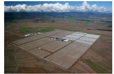
Thermal energy storage The Andasol CSP plant uses tanks of molten salt to store solar energy
