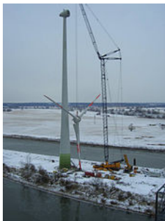
Erection of an Enercon E70-4 in Germany .
