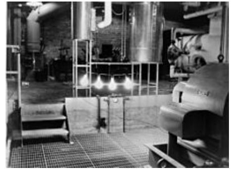
The first light bulbs ever lit by electricity generated by nuclear power at EBR-1 at Argonne National Laboratory-West, December 20, 1951.
