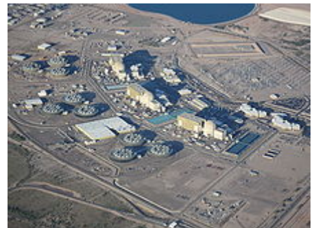
The Palo Verde Nuclear Generating Station, the largest in the US with 3 pressurized water reactors (PWRs), is situated in the Arizona desert. It uses sewage from cities as its cooling water in 9 squat mechanical draft cooling towers. [2][3] Its total spent fuel/"waste" inventory produced since 1986, is contained in dry cask storage cylinders located between the artificial body of water and the electrical switchyard.
