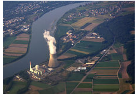
The 1200 MWe, Leibstadt fission-electric power station in Switzerland. The boiling water reactor (BWR), located inside the dome capped cylindrical structure, is dwarfed in size by its cooling tower. The station produces a yearly average of 25 million kilowatt-hours per day, sufficient to power a city the size of Boston. [1]
