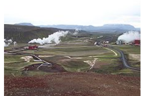
Krafla Geothermal Station in northeast Iceland
