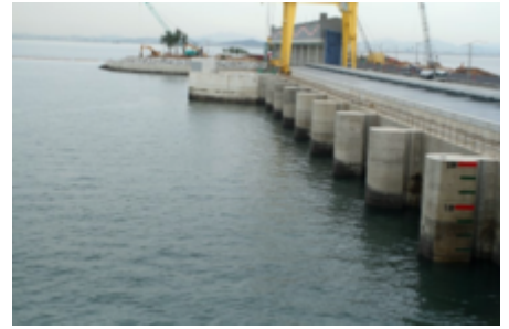
Sihwa Lake Tidal Power Station, located in Gyeonggi Province, South Korea, is the world's largest tidal power installation, with a total power output capacity of 254 MW
