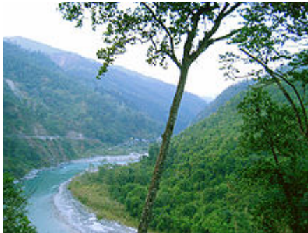
National Highway 31A winds along the banks of the Teesta River near Kalimpong (West Bengal), in the Darjeeling Himalayan hill region.
