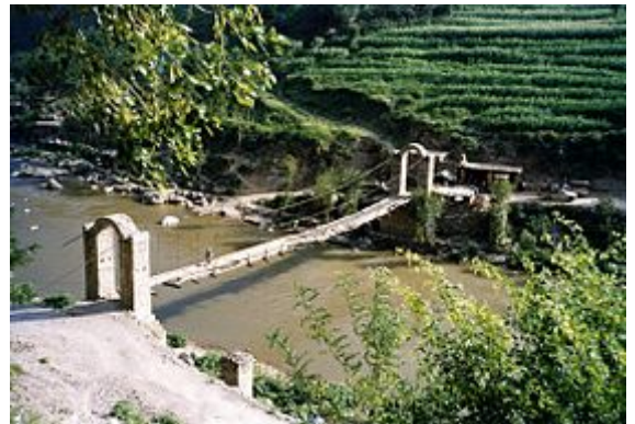
Footbridge on the Indus River in Pakistan
