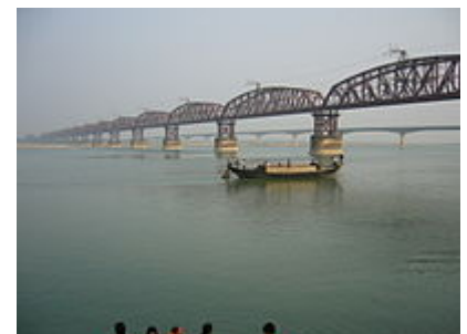
Hardinge Bridge, Bangladesh, crosses the Ganges-Padma River. It is one of the key sites for measuring streamflow and discharge on the lower Ganges.
