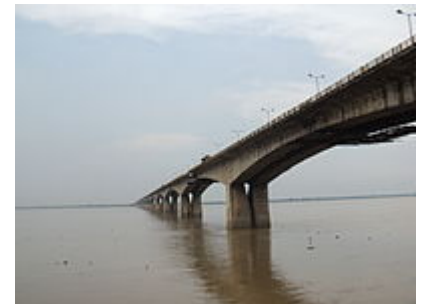
The Mahatma Gandhi Setubridge over the Ganges connecting the cities of Patna and Hajipur
