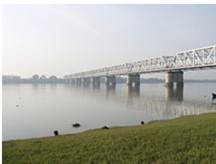
Railway Bridge on river Narmada at Bharuch, Gujarat
