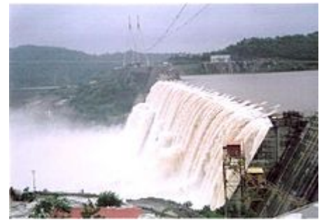
Sardar Sarovar Dam Gujarat, partially completed (up to E.L.121.92 m)
