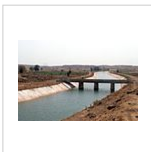
Sardar Sarovar Canal at with flow
