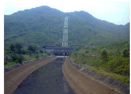
Upper Indravati power house
