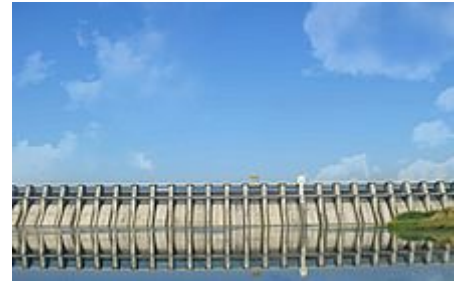
An upstream view of Jayakwadi Dam.
