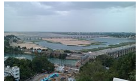
Down stream view of Prakasam Barrage.
