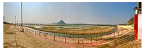
Panorama of Prakasam Barrage and Railway bridges on Krishna near Vijayawada
