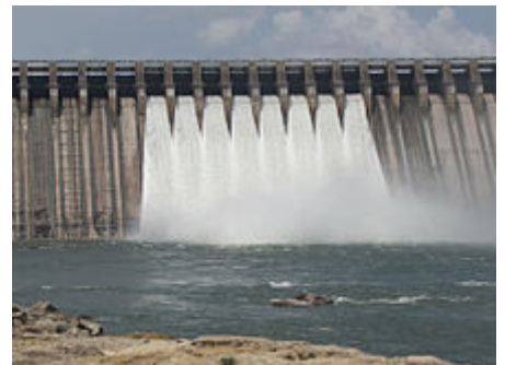
Nagarjuna Sagar Dam Gates view
