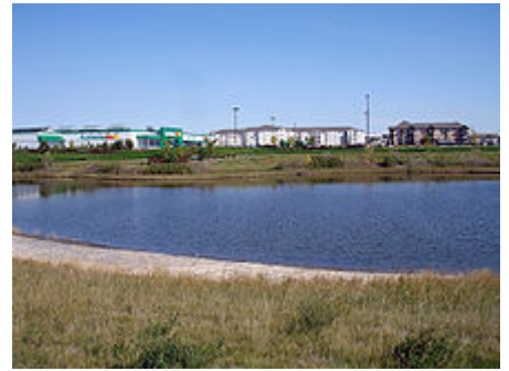
Retention basin for controlling urban runoff
