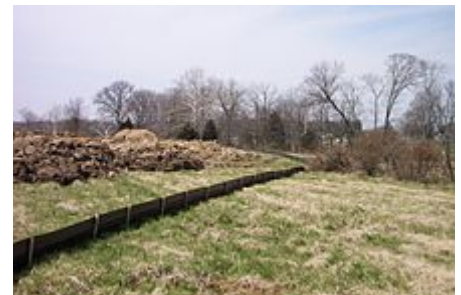
Silt fence installed on a construction site.
