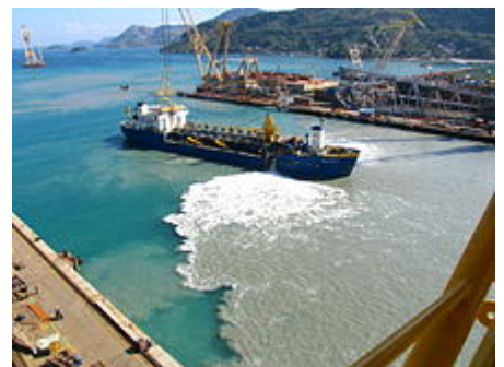
Point source pollution at shipyard in Rio de Janeiro, Brazil.
