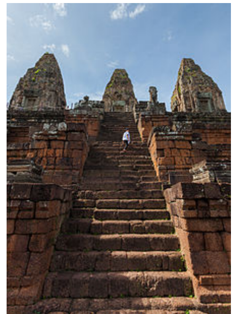
Example of construction with laterite in Pre Rup, Angkor, Cambodia.
