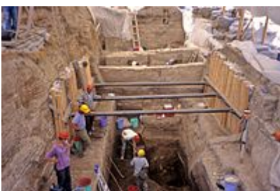
Deep trenches in the site
