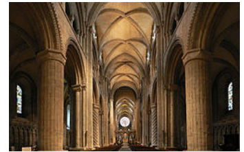
The transition from Romanesque to Gothic styles is visible at the Durham Cathedral in England, where both pointed and round arches are used in the cathedral's design.
