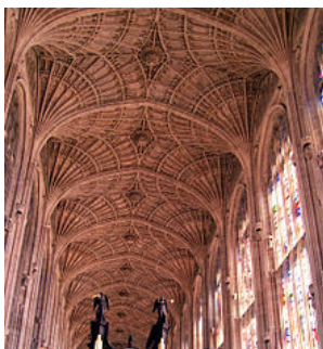
The depressed arch supported by fan vaulting at King's College Chapel, England.
