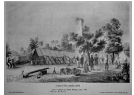
Measurement of the Calcutta baseline in 1832 based on a sketch by James Prinsep. This shows surveyors stretching a chain on coffers supported on pickets. The chain is housed under shade to reduce errors due to thermal expansion, and is aligned using a boning telescope.
