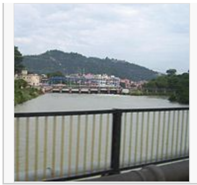
Photograph (2008) of the head works of the Ganges Canal in Haridwar, viewed from the opposite side.
