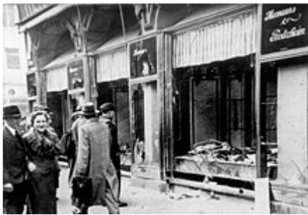
Damage caused during Kristallnacht , 9 November 1938
