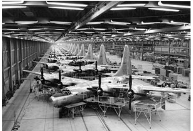
Mass production of Consolidated B-32 Dominator airplanes at Consolidated Aircraft Plant No. 4, near Fort Worth, Texas, during World War II.
