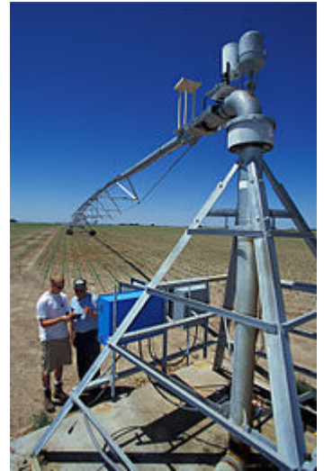
The hub of a center-pivot irrigation system
