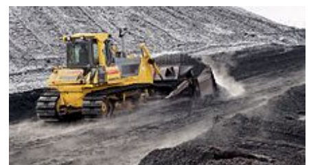
Komatsu bulldozer pushing coal in Ljubljana Power Station
