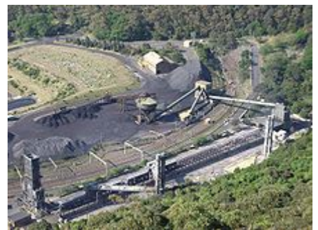
The Illawarra Coke Company (ICC) in Coalcliff, New South Wales, Australia.
