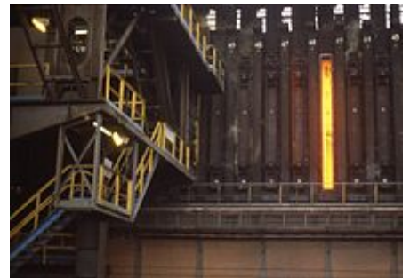
Coke oven at smokeless fuel plant, Abercwmboi, South Wales, 1976
