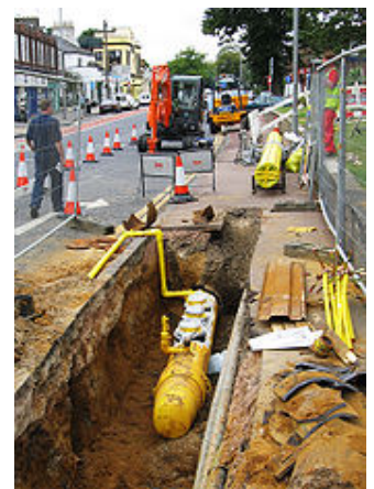
Polyethylene plastic main being placed in a trench.
