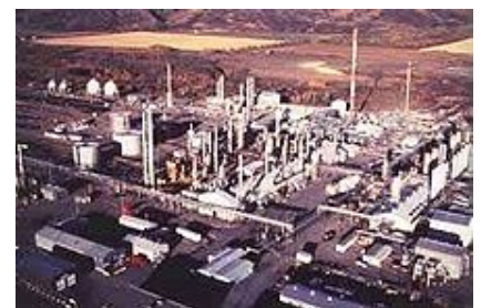
The McMahon natural gas processing plant in Taylor, British Columbia, Canada. [36]
