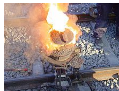
Thermite reaction proceeding in railway welding. Shortly after this, the liquid iron flows into the mould around the rail gap
