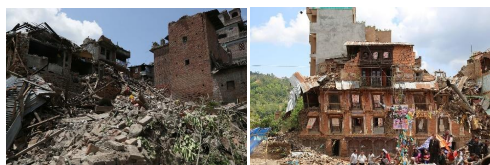
Pics: Nepal/Gorkha Earthquake destruction
