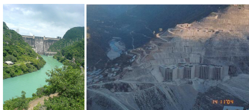
Pics: Bhakra-Nangal dam & Tehri dam
